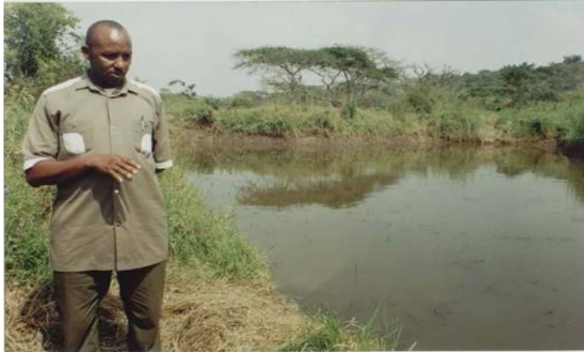
Figure 6 (b). Valley tank rehabilitated with DHP support
